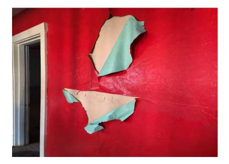
Photo illustrates potential lead based paint peeling on the walls of the upper level of the building.
